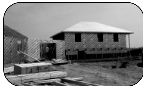
COMING SOON: Varency Home, under construction. Photo by Bruce Barrett
